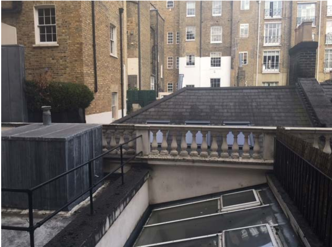
Rear of building, existing lean-to roof
